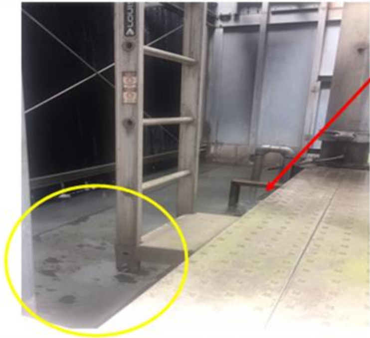
Figure 5: The sample should be collected by the door, inside the basin (yellow circle). Red arrow indicates the most turbulent part of the basin.
